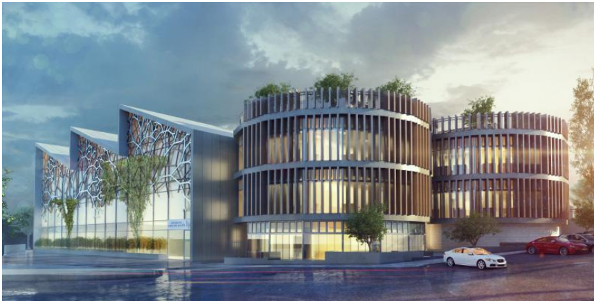
Shenkar College - Under Construction (2015-2017)
